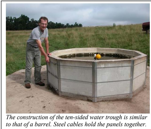
*The construction of the ten-sided water trough is similar to that of a barrel. Steel cables hold the panels together.*
