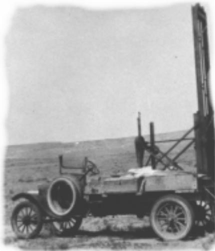
*Some soil scientists used this rig in 1927 to save the backbreaking work of an auger.*
