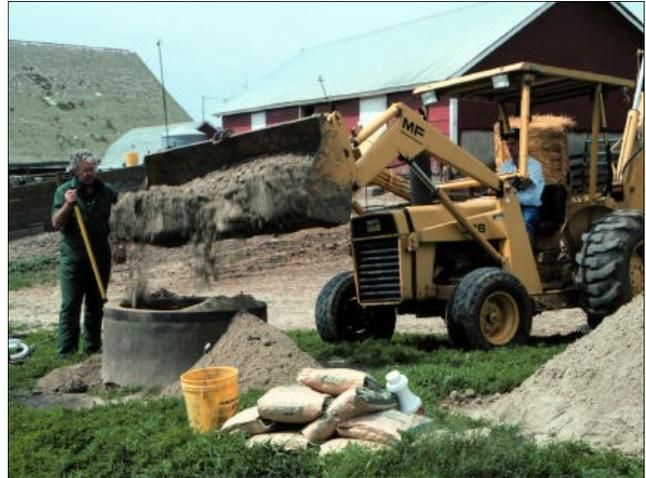
be sealed with material that will prevent surface water from entering the wellhead and the soils around the wellhead will be graded to prevent ponding.
